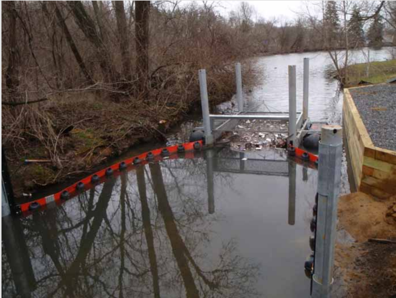
Duck Pond inflow channel trash rack
