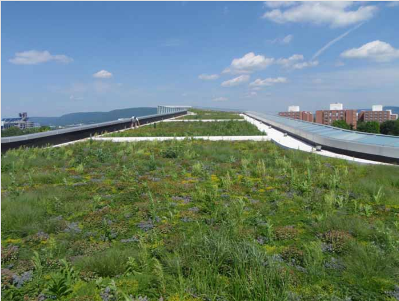
Katz Law School Building Roof
